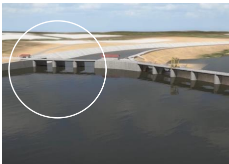
Computer-generated Image of the Water Intake (circled zone) of the Headrace canal
