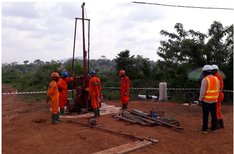
Bouygues Energie & Services and Africa Geoproject teams on a drilling site
